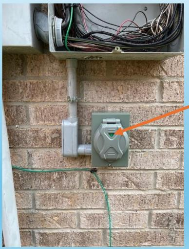
50AMP connection from Generator To House Main Panel. **Green light** On connector lights when Generator is Supplying Power.
