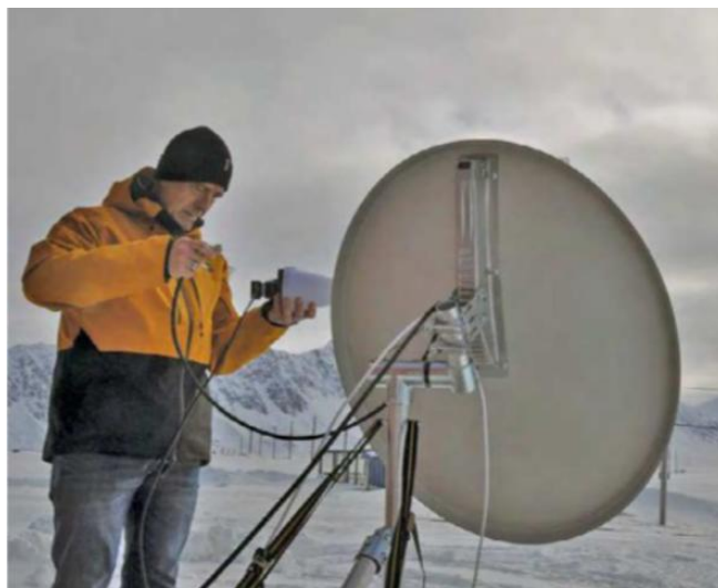
Patrick Blancquaert, ON4DCU, during the installation of the Triax satellite antennas. The team brought two 120-centimeter antennas because they were active with two stations at the same time on the QO-100 satellite.
