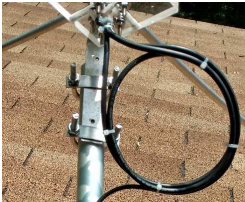
Figure 5 — A close-up view of the feed system with the turnstile mounted in place.
